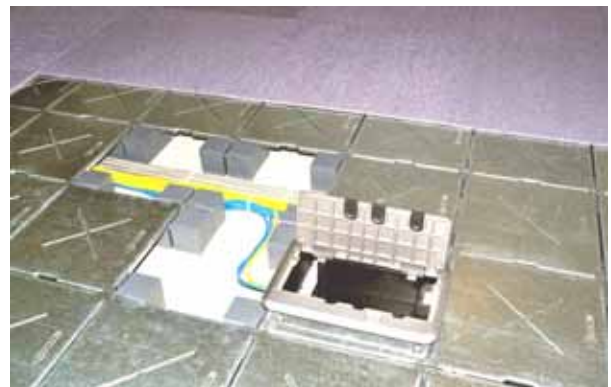
Netfloor SB603 installed by replacing one Top-Panel, facilitates 2 power sockets, 3 data jacks.
