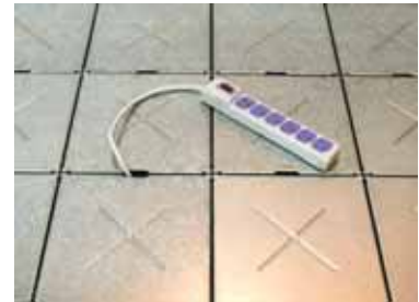
Power and data extension from the junction box under Top-Panel
