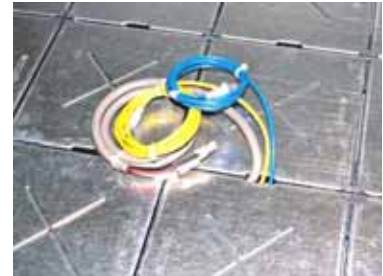
Cables extended through the cable-exit
